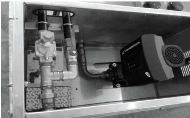
Water intake group. Solenoid valve and float valve for manual filling. Water supply 1" 1/4 GAS female outlet.
