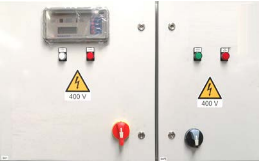
MAIN ELECTRICAL PANEL AND ADIABATIC ELECTRICAL PANEL
