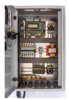
Metal casing painted with RAL7035, 120 micron thickness, suitable for outdoors installation. Protection class IP65.
